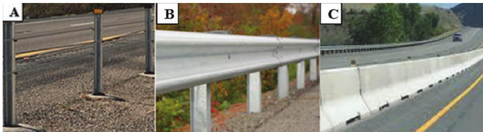
Figure 3: Longitudinal Barrier: Flexible Barriers (A); Semirigid Barriers (B); and Rigid Barriers (C)
